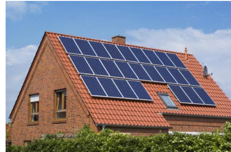
Residential Rooftop Solar
